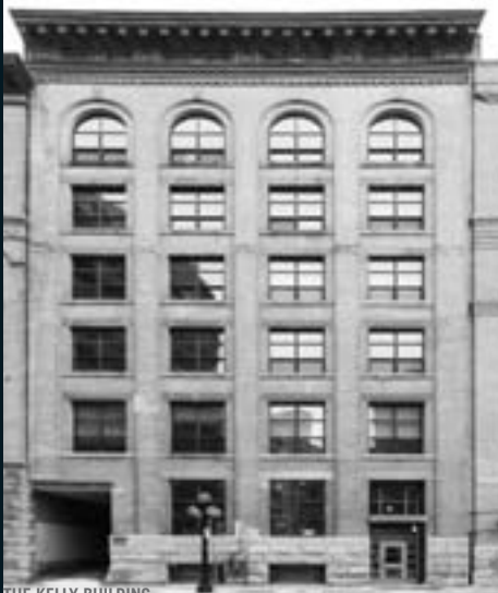
THE KELLY BUILDING
