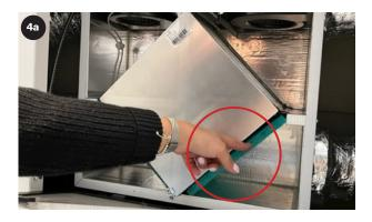
If the filters are in this condition, vacuum only and then go to Step 5.
